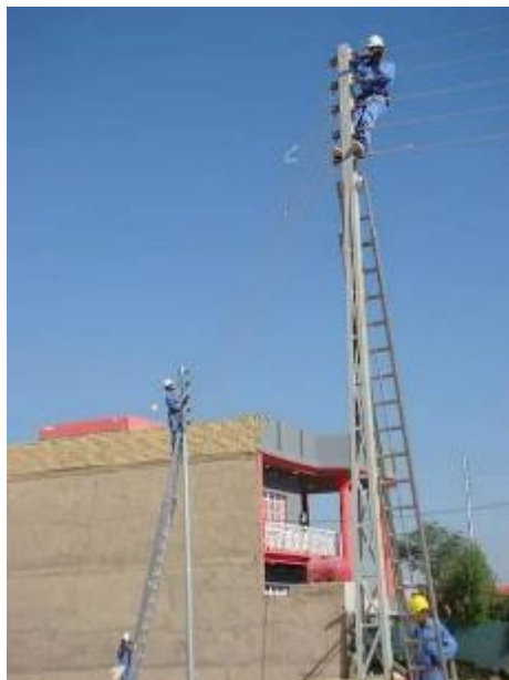
Figure 3-15 Erecting Lattice and Tubular Steel Poles in Previuos Projects in Mosul, Iraq
